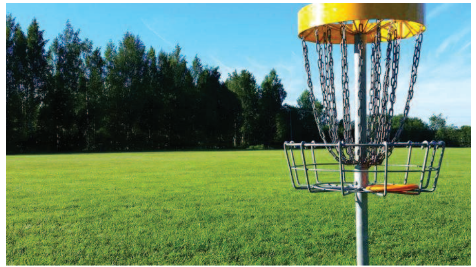
Alton-Godfrey Rotary Club Members make a difference. Temperatures in the 90s did not deter members who gathered at LaVista Park in Godfrey to install new disc golf tees at the park.
